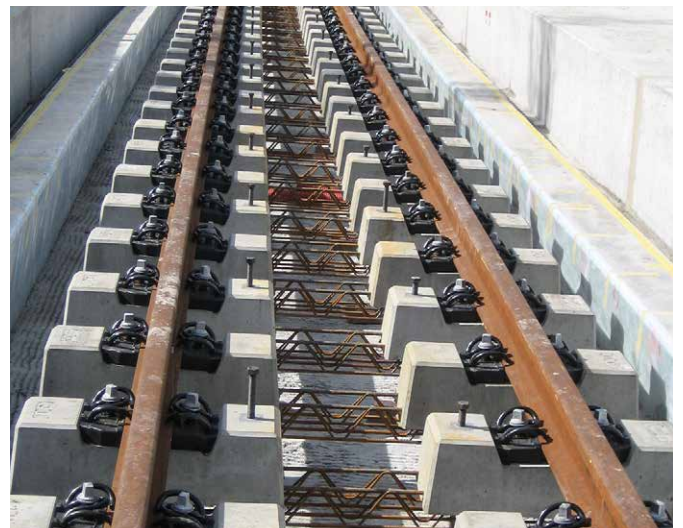
RHEDA CITY open formation track installation in Samedan, Switzerland.
